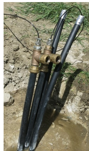
Figure 2: a) Position of the optical cables inside the U pipe BHE; b) The optical cables installed inside the U pipe
